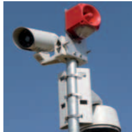
FLIR Systems SR-Series thermal imaging camera, a sound and light beacon and a CCTV dome installed at an observation point.
